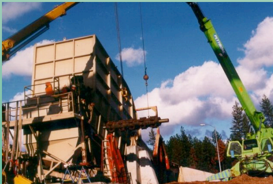
Headshaft on Reclaimer Mt. Burney, CA
